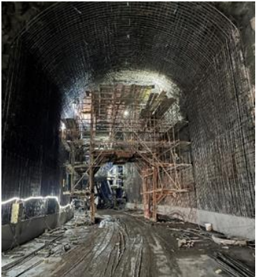
Upstream Entrance Reinforcement Work
