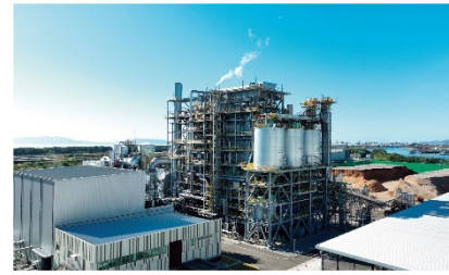
Hirohata Biomass Power Plant (Hyogo Prefecture)
