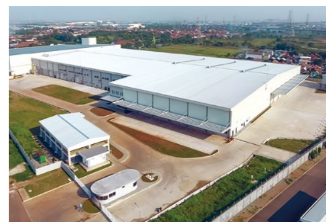
Panoramic view of the new plant
