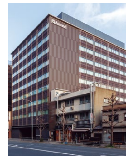
OVOL Kyoto Ekimae Building
