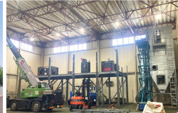
Plant installation work
