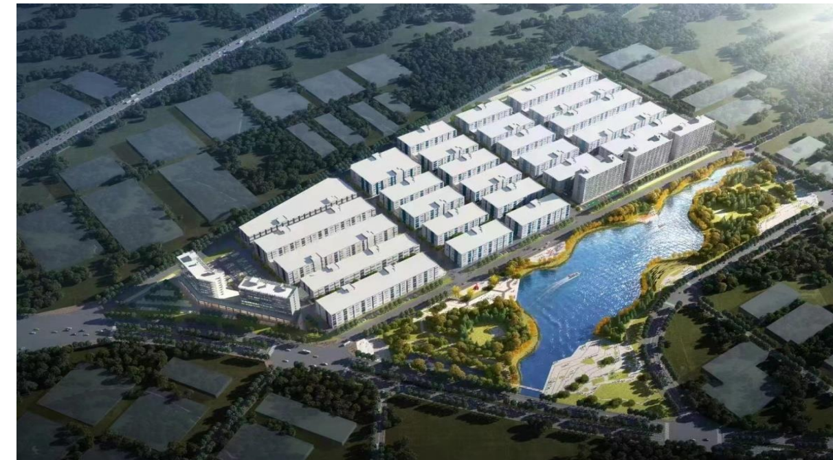
Mar 2023 Shunde Daliang new factory completed
