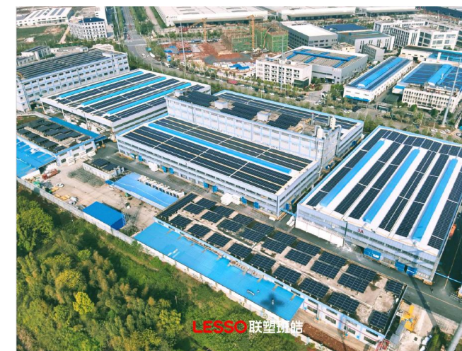
Solar Panel Installation Example
