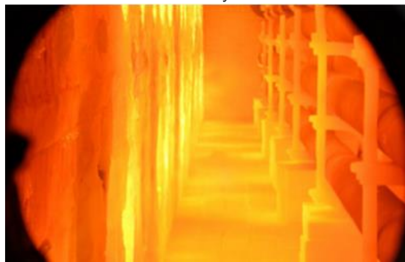
Inside the naphtha cracking furnace during ammonia combustion
