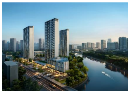
▲ Wenzhou Ouhai Project (Completed in 2024)
