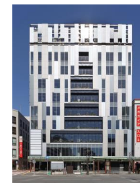
▲ FUNDES Kamata (Completed in March 2024)
