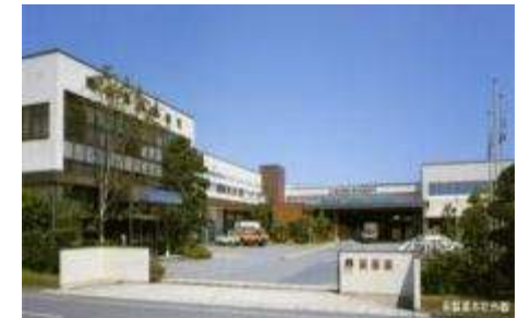
Kotobuki Seika Co., Ltd., Main Plant
