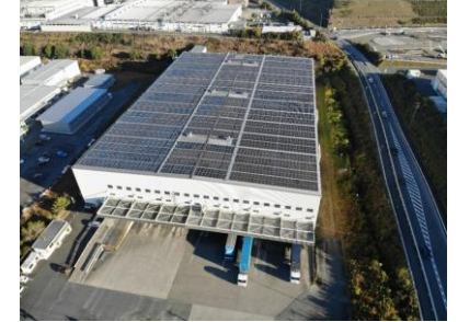
Solar panel power generation system on roof of Shinshiro-Minami Plant
