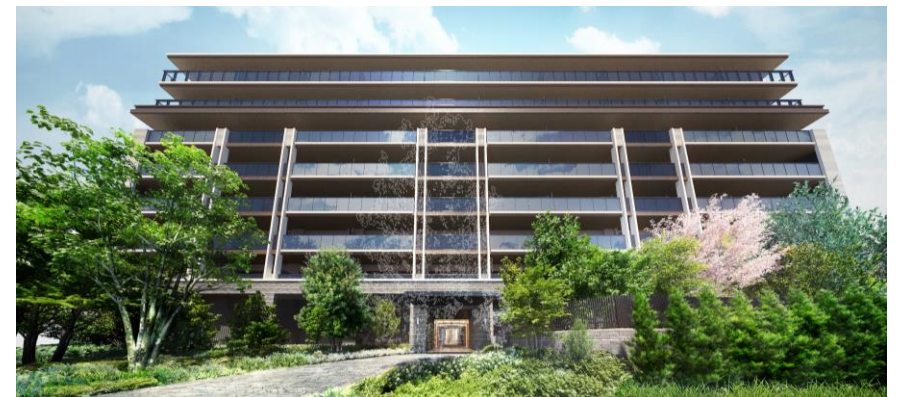
DUO SCENE Saitama South (Warabi City, Saitama, 112 units, to be delivered in March 2025)
