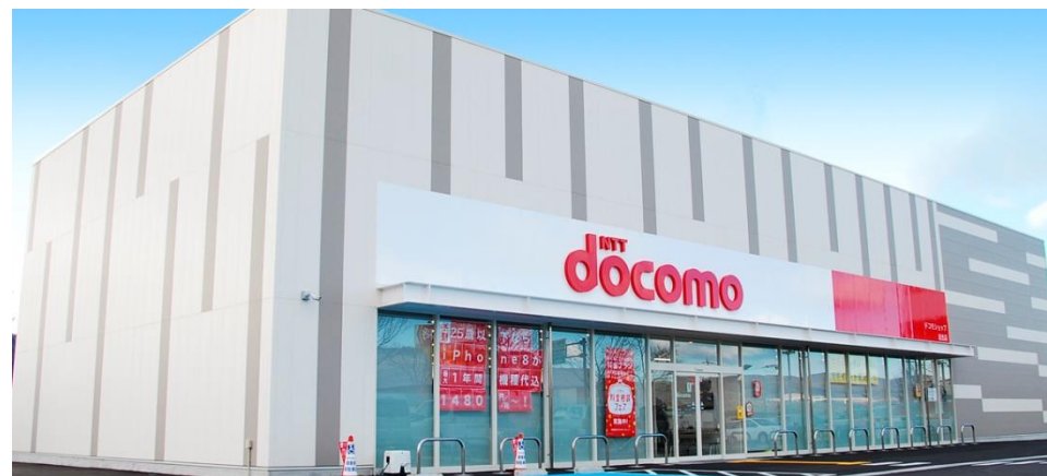
Iwade Store (largest store in Wakayama Prefecture)
