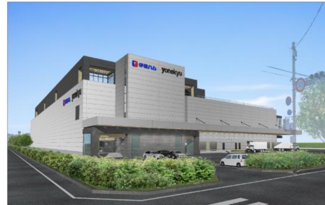
Exterior image of new Mishima Plant
