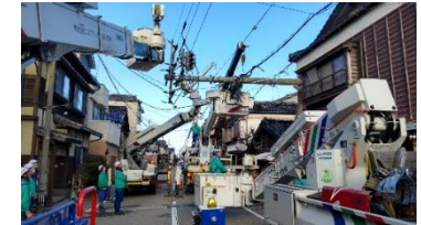
Repair of broken poles
