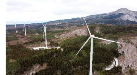
【Green Power Fukaura】 Output 73,600kW (Operation Started : Feb.2024)
