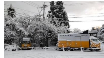
Emergency power transmission by high-voltage generator truck
