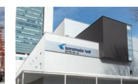
Kanamoto Hall (Sapporo Civic Hall) Housing a Large 1,500-person Event Hall as well as Small, Medium and Large Conference Rooms
