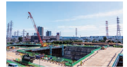
Kanagawa Prefecture Station (tentative name) of the Linear Chuo Shinkansen under construction
