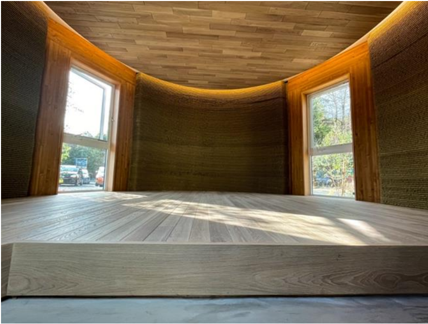
3D-printed housing Lib Earth House “modelA” (Construction site: Yamaga City, Kumamoto Prefecture)
