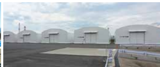
2023 Land leveling work is completed
