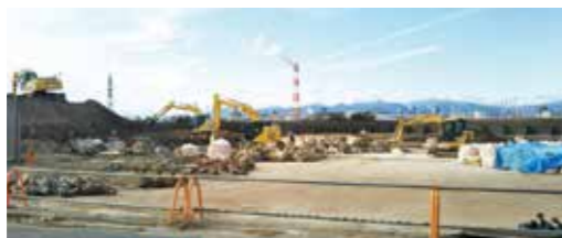
2018 Removal work is underway
