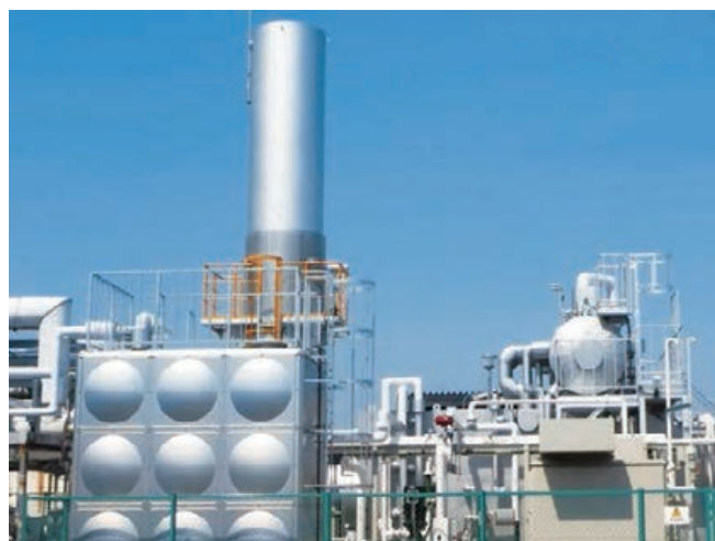
New co-generation power system (Japan)
