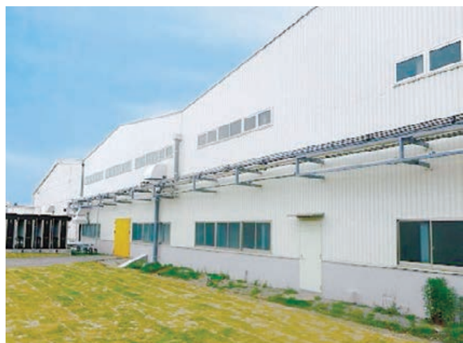
Production facilities for hollow fiber membrane modules (Japan)
