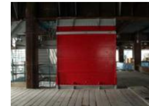
Viscous seismic damping wall
