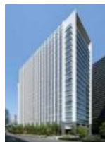
ARK Hills South Tower
