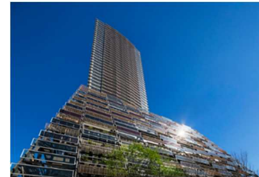
Brillia Tower Ikebukuro (completed in 2015) Japan's first large-scale complex tower residence (49 floors, 432 units) integrated with a ward government building. 1st-10th floors: Toshima Ward Office, commercial facilities, etc. 11th-49th floors: Residential
