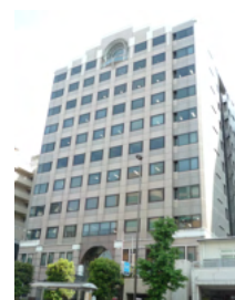
Narimasu Tosei Building
