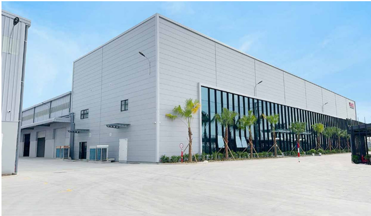
VSUN Ingot and Wafer Plant
