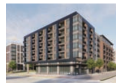
Total Project Cost: 21.3 billion yen
