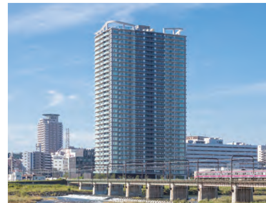
Brillia Tower Seiseki Sakuragaoka BLOOMING RESIDENCE (Completed in 2022)
