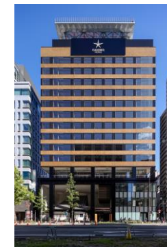
▲ Candeo Hotels Osaka Shinsaibashi (Completed in 2023)
