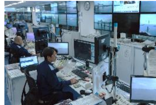
TOKYO WAN Vessel Traffic Service Center of the Japan Coast Guard, where our Vessel Traffic Services system is installed
