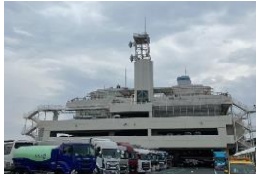
Maritime surveillance radar installed at the Umihotaru Parking Area in Tokyo Bay
