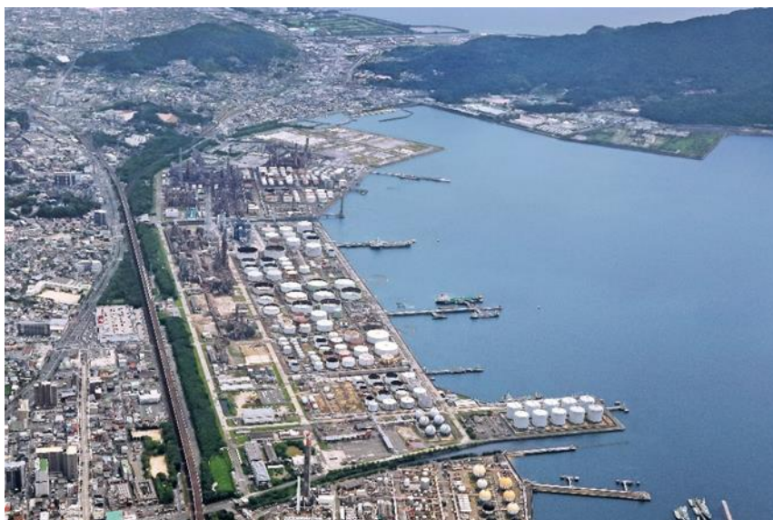
Tokuyama Complex, the planned construction site of the HEFA-SAF production facility (center of photo)
