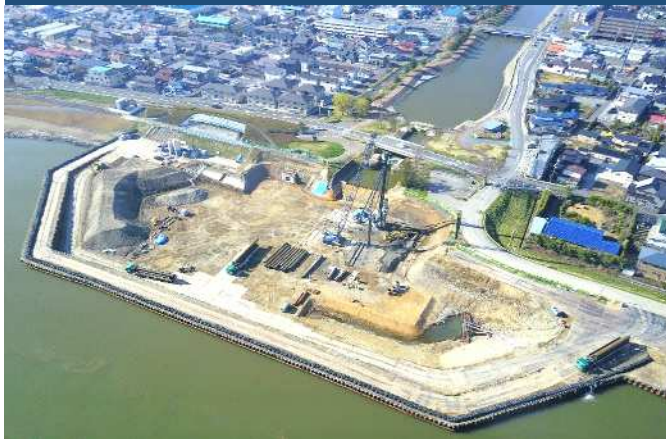
Wind and flood damage countermeasure works
