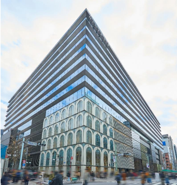
Arranged in March 2024 One of the largest project to date
